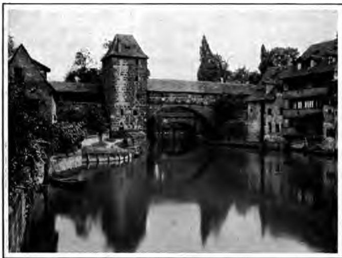
22. THE PEGNITZ AT NUREMBERG. — Notice the fortifications and the way the wall with its covered passage is carried over the river.
